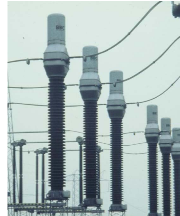
Plate 5.15 – Typical Current Transformer Image: ©ABB
